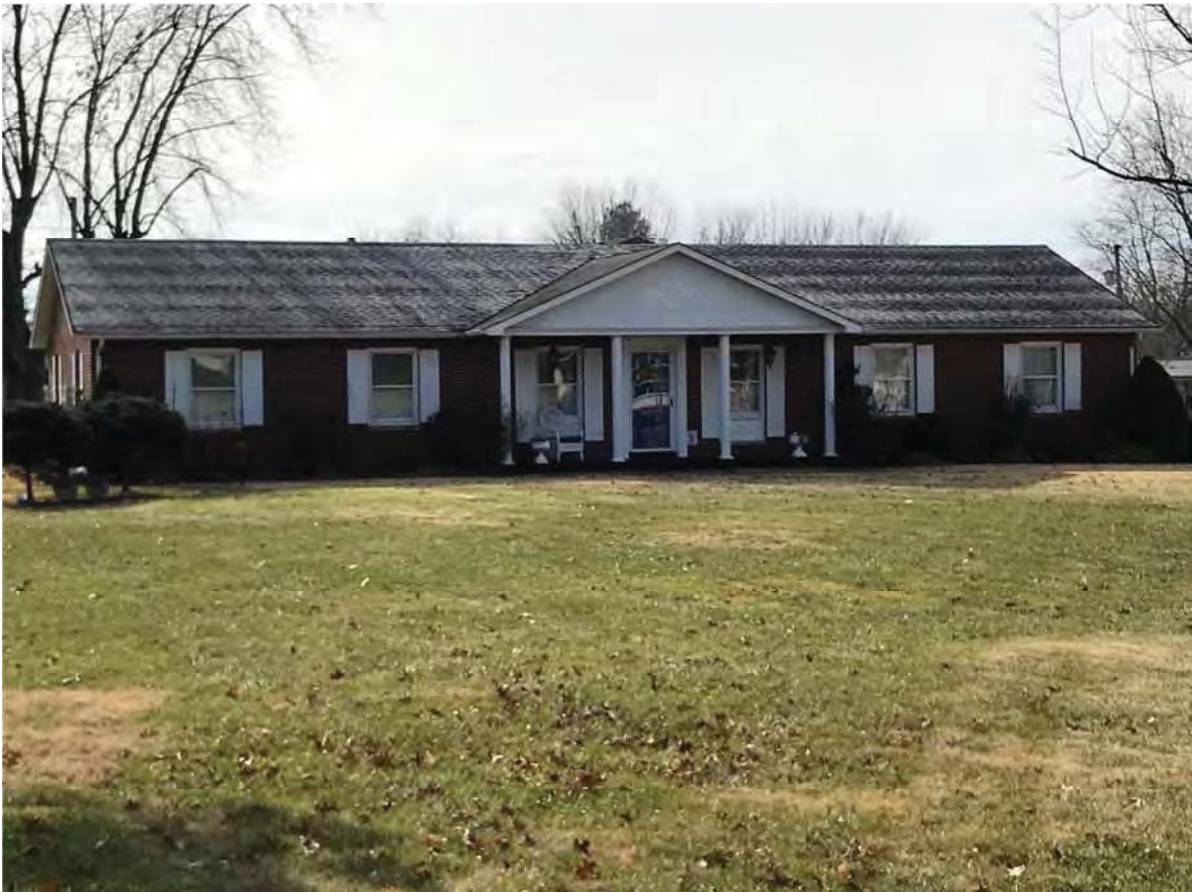
64. Looking SSW at Lochmueller #16, Contributing, 1841 Highway 54 East
