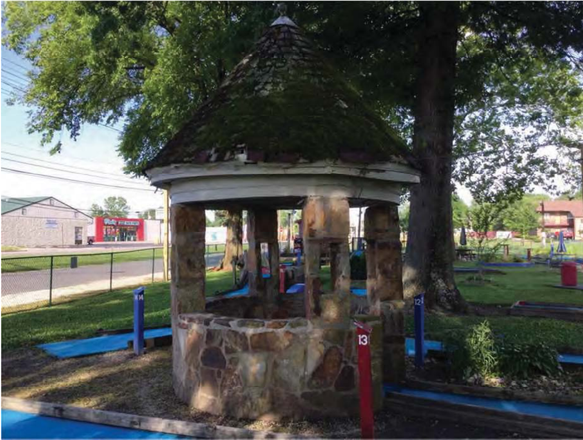
5. Looking SW at stone shelter in miniature golf course in Humphreys Park, IHSSI #055-362-27020, Notable, National Register-eligible
