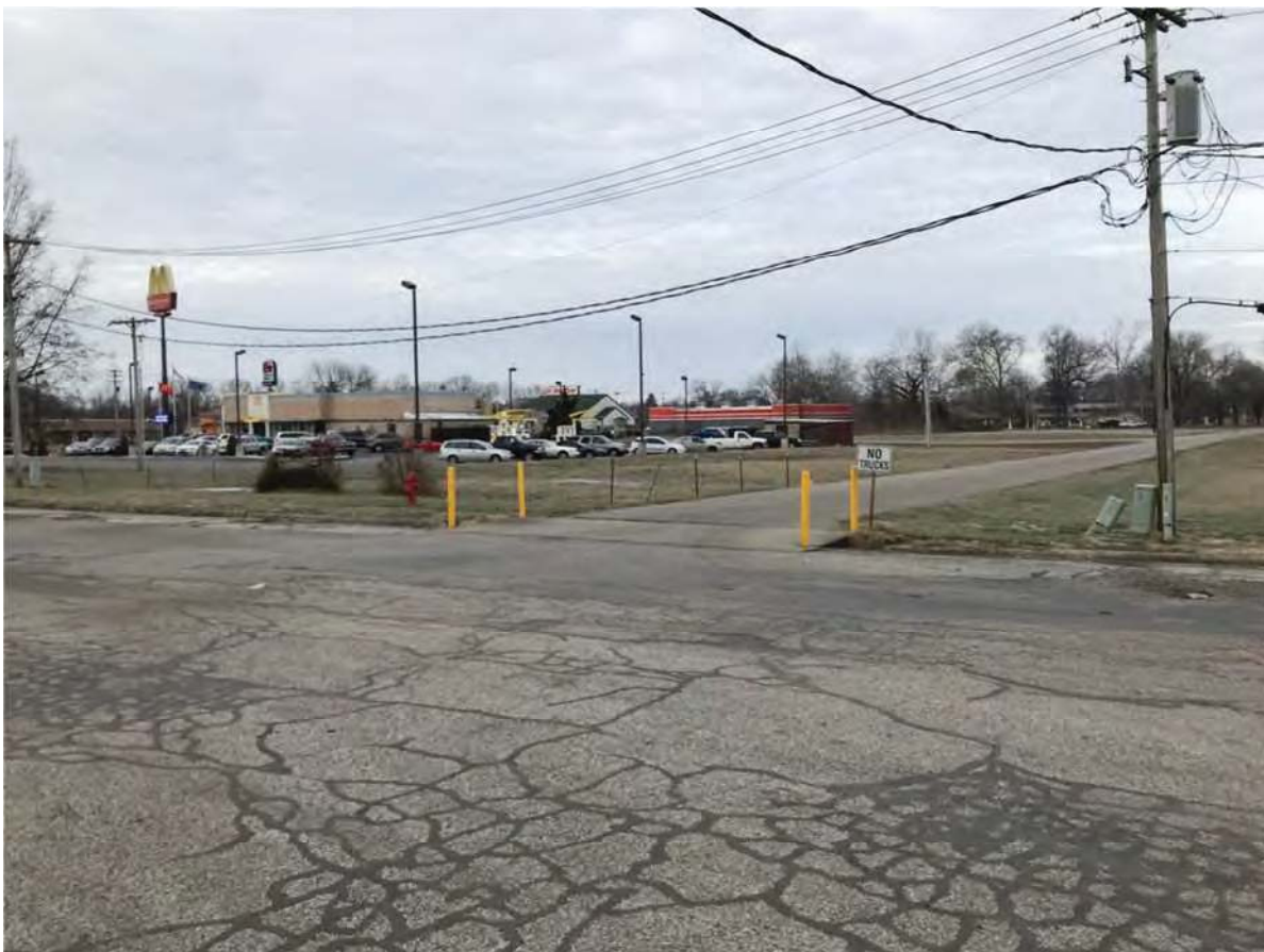
30. Looking SW at access drive entrance to Linton Shopping Center
