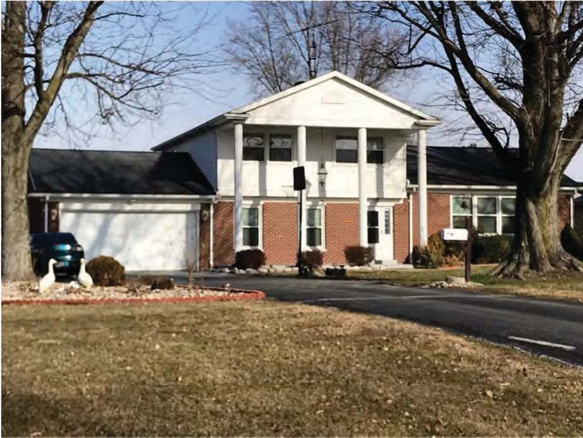
53. Looking NE at Lochmueller #9, Contributing, 1760 Highway 54 East
