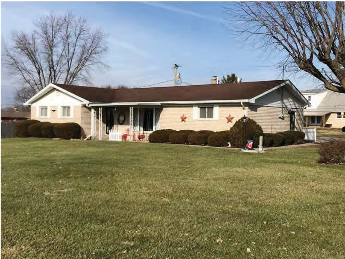
56. Looking NW at Lochmueller #12, Contributing, 1780 Highway 54 East
