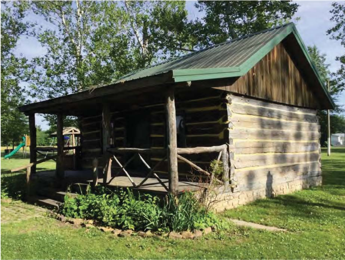
11. Looking NW at log cabin in Humphreys Park, IHSSI #055-362-27020, Notable, National Register-eligible
