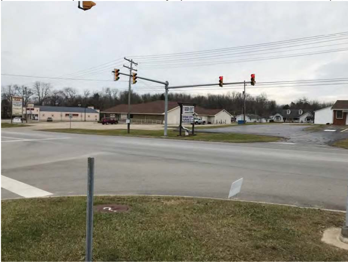
85. Looking NW at the intersection of Highway 54 and Goody's clothing store access drive
