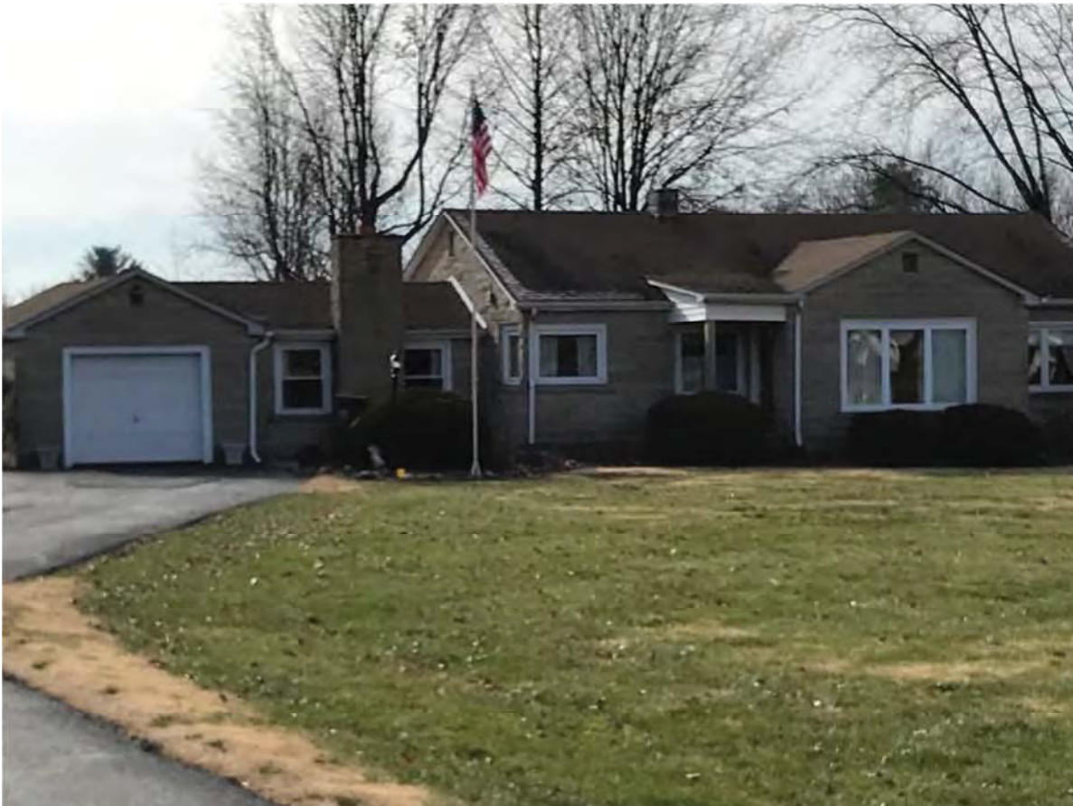
66. Looking SSW at Lochmueller #18, Contributing, 1861 Highway 54 East
