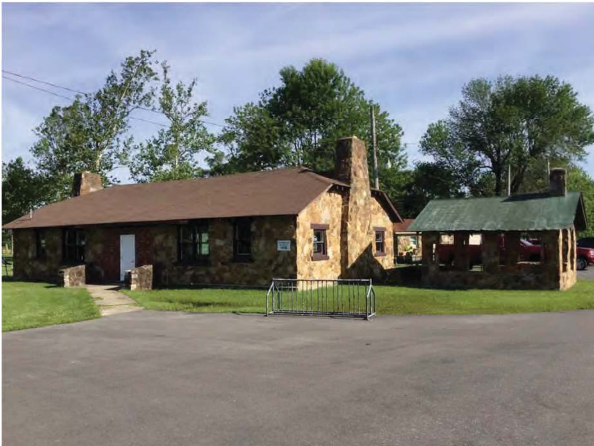
14. Looking NW at stone park building with adjacent stone hearth shelter in Humphreys Park, IHSSI #055-362-27020, Notable, National Register-eligible
