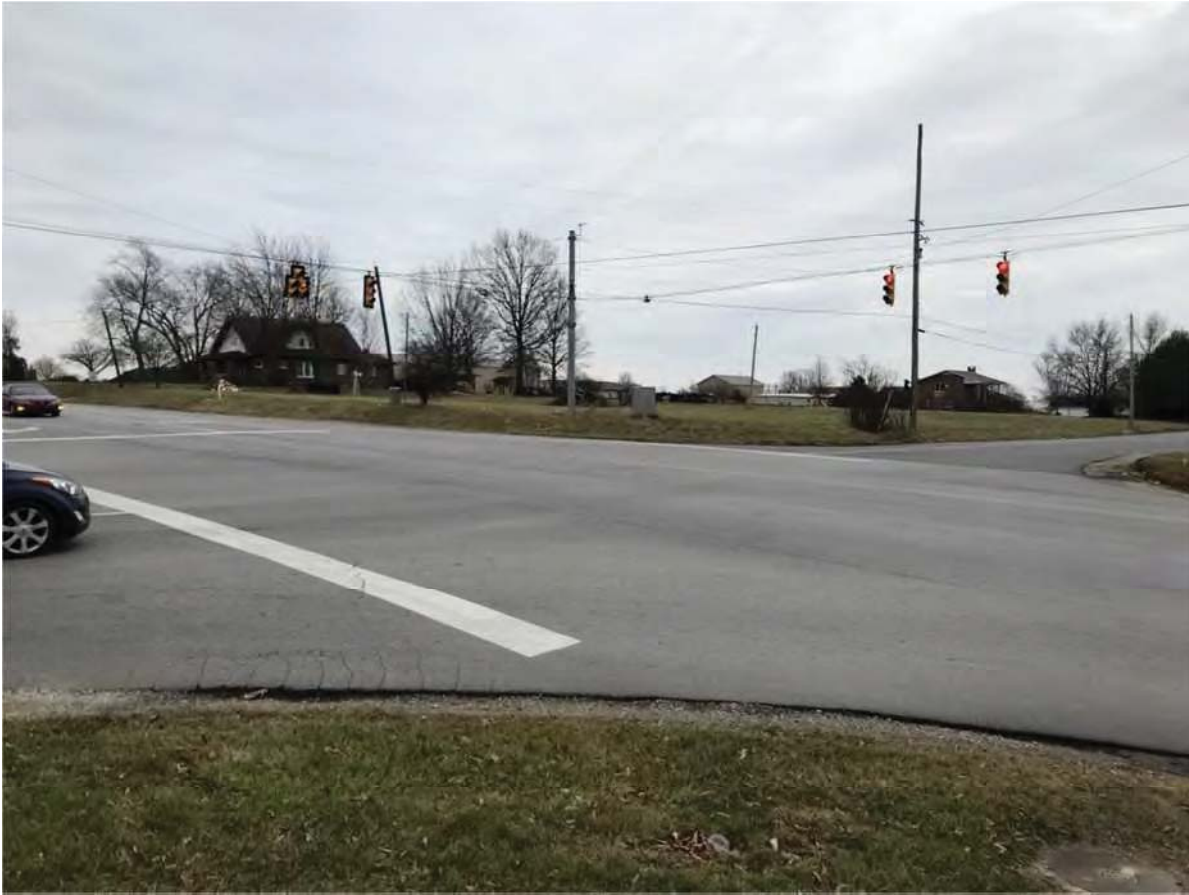
95. Looking SE at the intersection of Highway 54 and CR 1000 W
