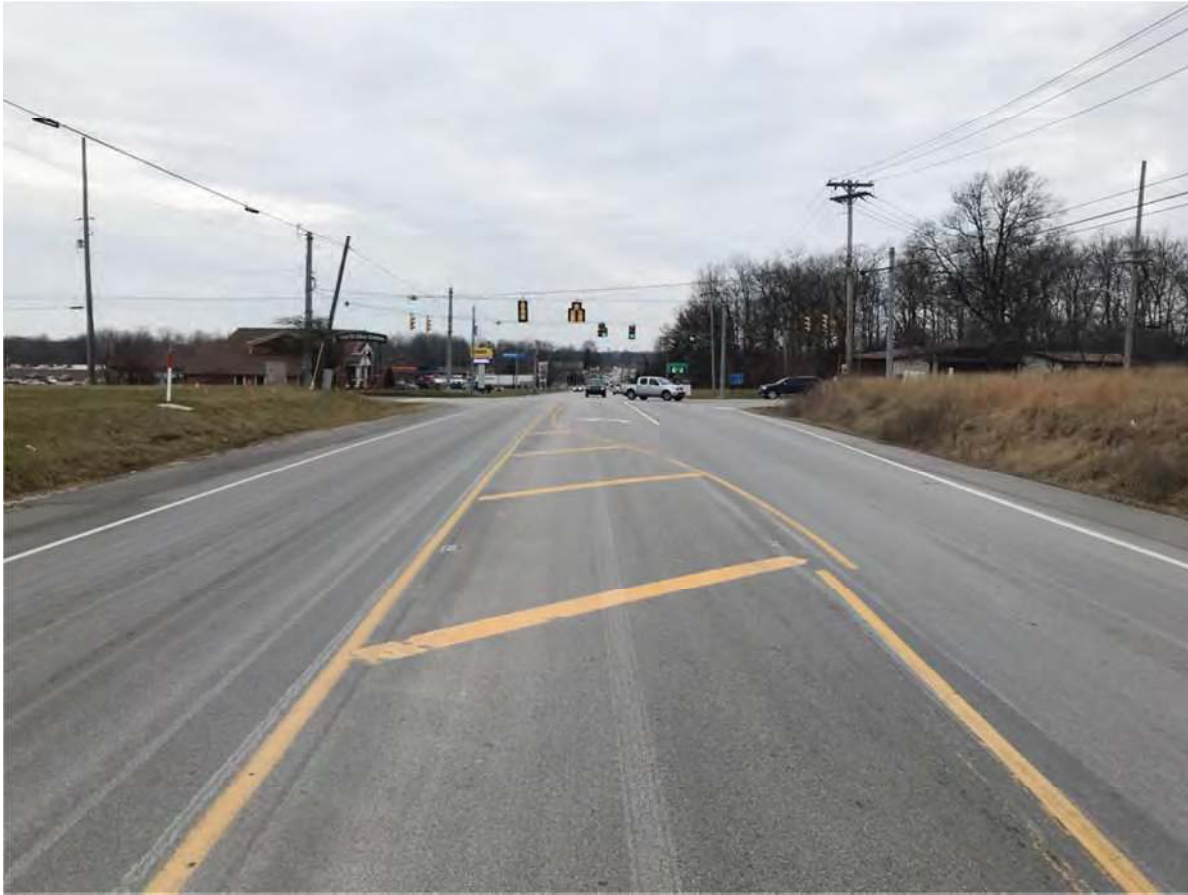
99. Looking W from E end of APE on Highway 54
