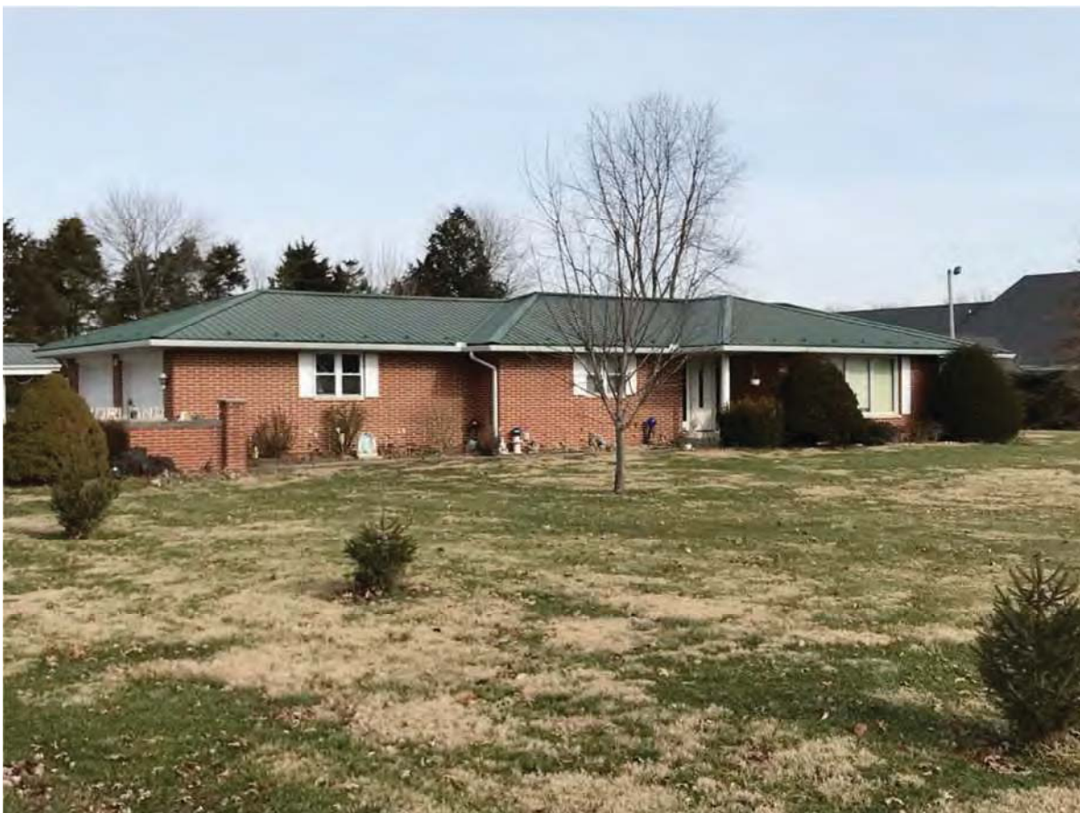
74. Looking NE at Lochmueller #21, Contributing, 1910 Highway 54 East
