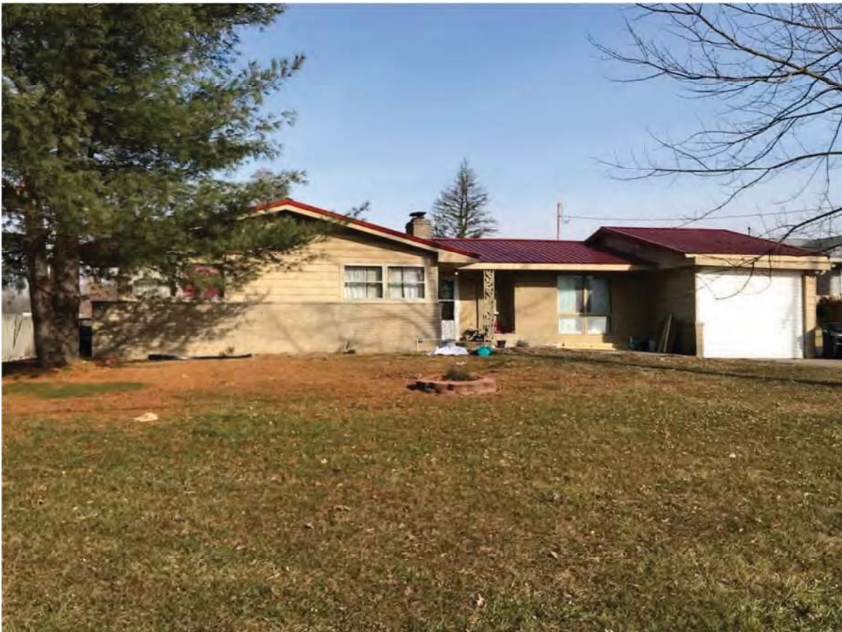
48. Looking NE at Lochmueller #4, Contributing, 1720 Highway 54 East
