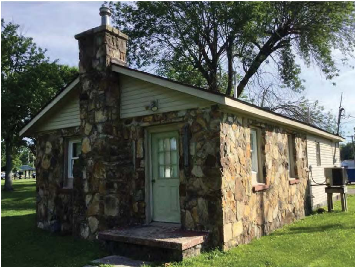
16. Looking NE at stone park building with frame addition in Humphreys Park, IHSSI #055-362-27020, Notable, National Register-eligible
