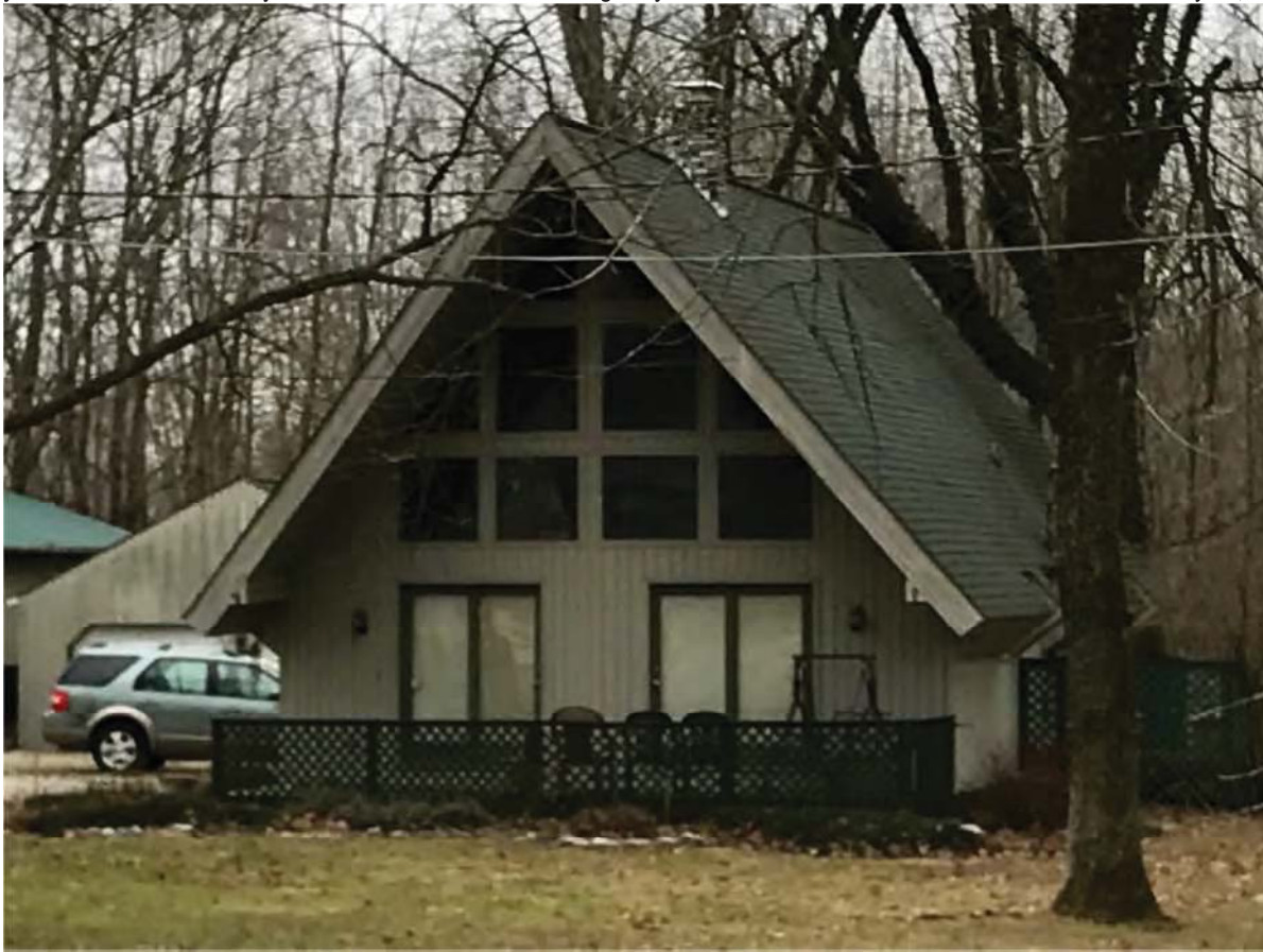
81. Looking SSE at Lochmueller #26, Contributing, 2105 Highway 54 East
