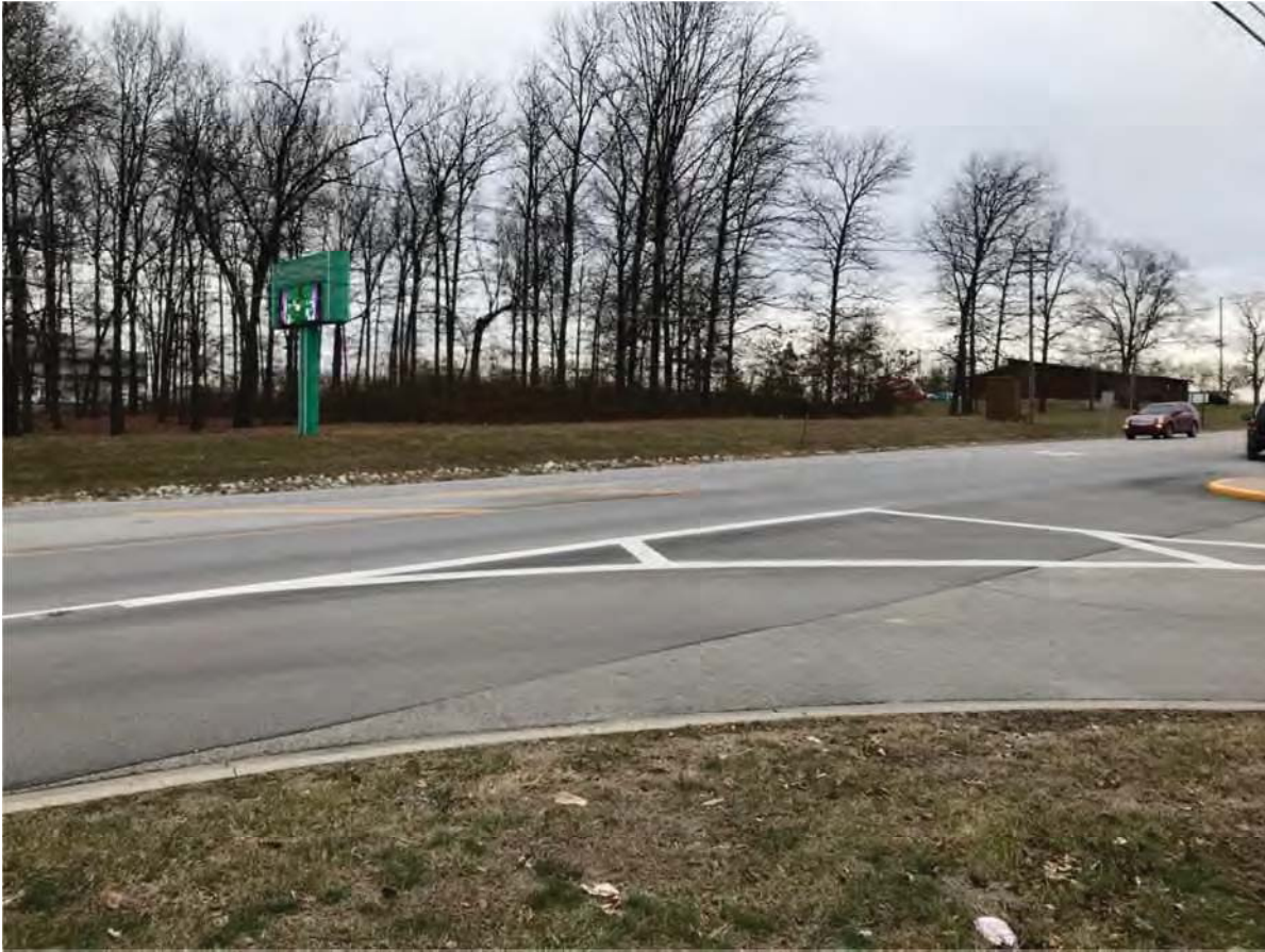
87. Looking NE at the intersection of Highway 54 and Walmart access drive
