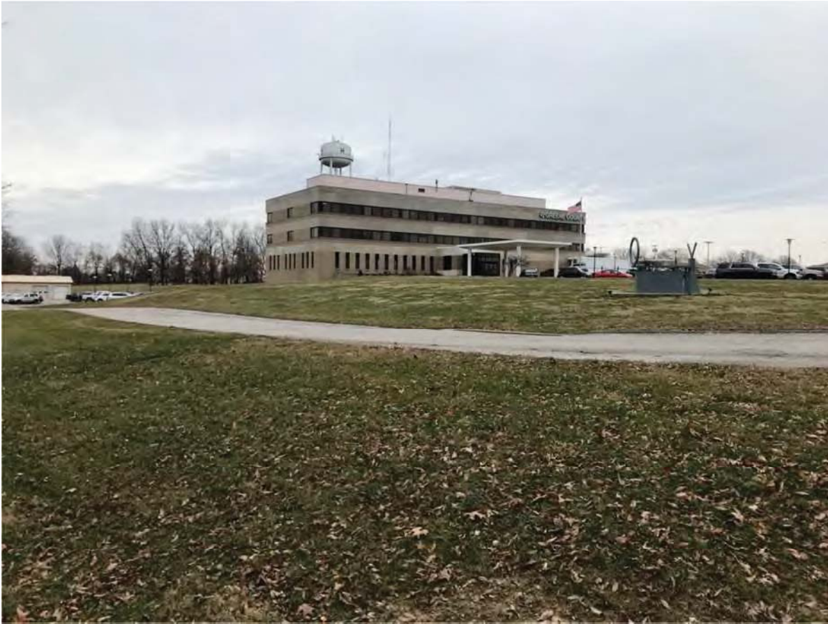
93. Looking NE at Greene County General Hospital, trail will end at this hospital
