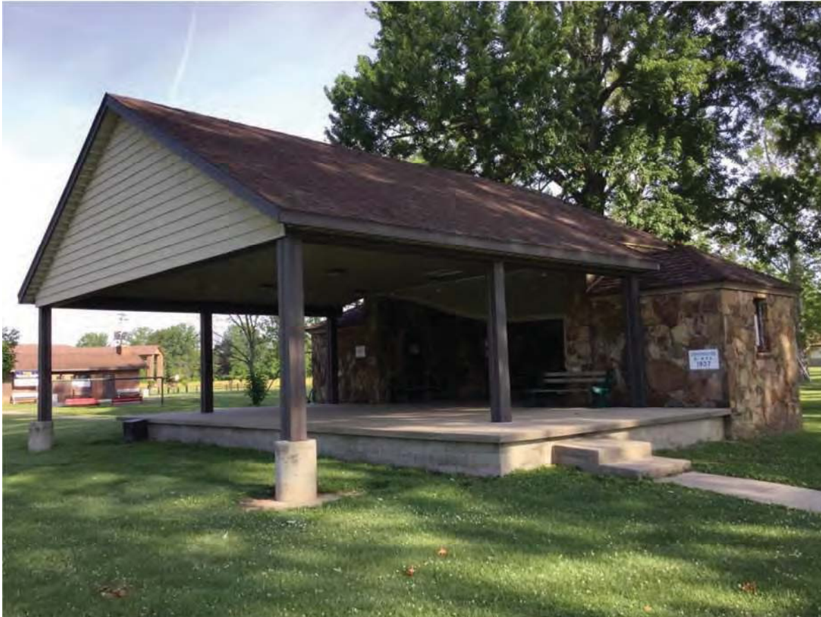
7. Looking NW at stone bandstand shelter in Humphreys Park, IHSSI #055-362-27020, Notable, National Register-eligible
