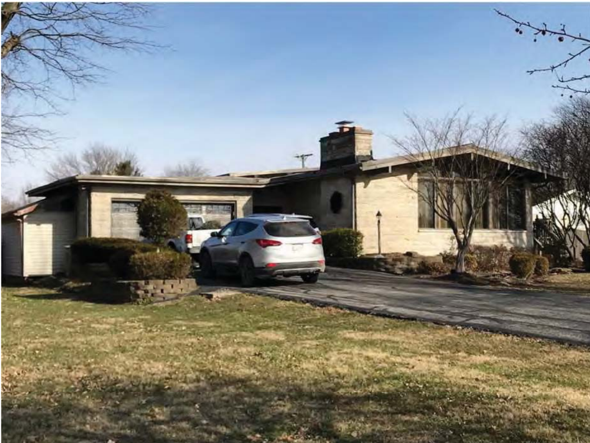
54. Looking NE at Lochmueller #10, Contributing, 1770 Highway 54 East
