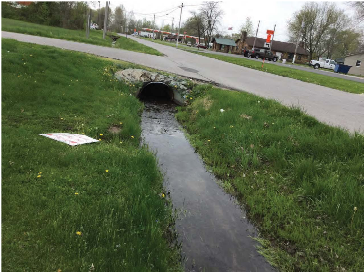
4. Looking south (downstream) UNT 2 towards culvert to be extended
