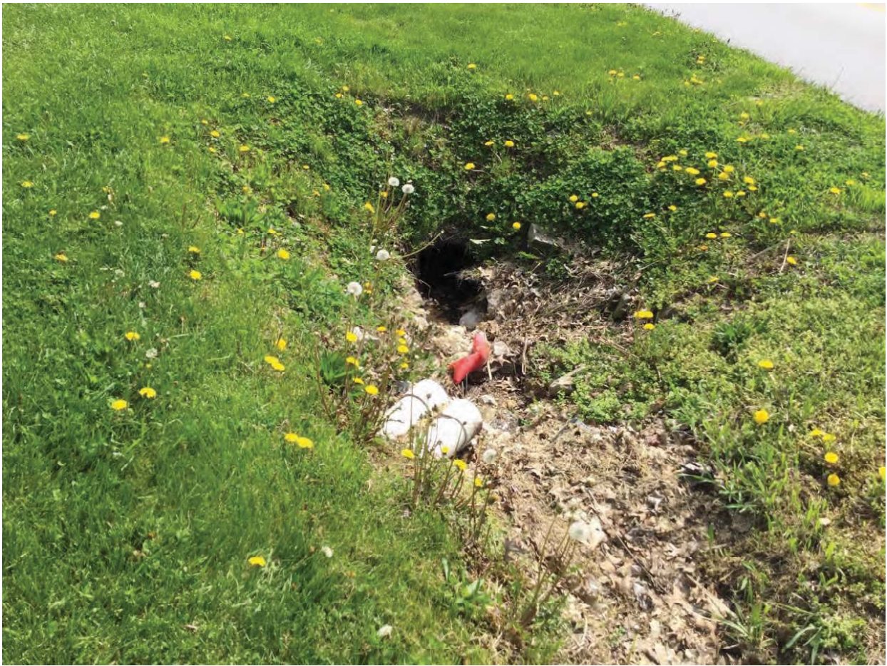
25. Looking east towards culvert at the end of UNT 3
