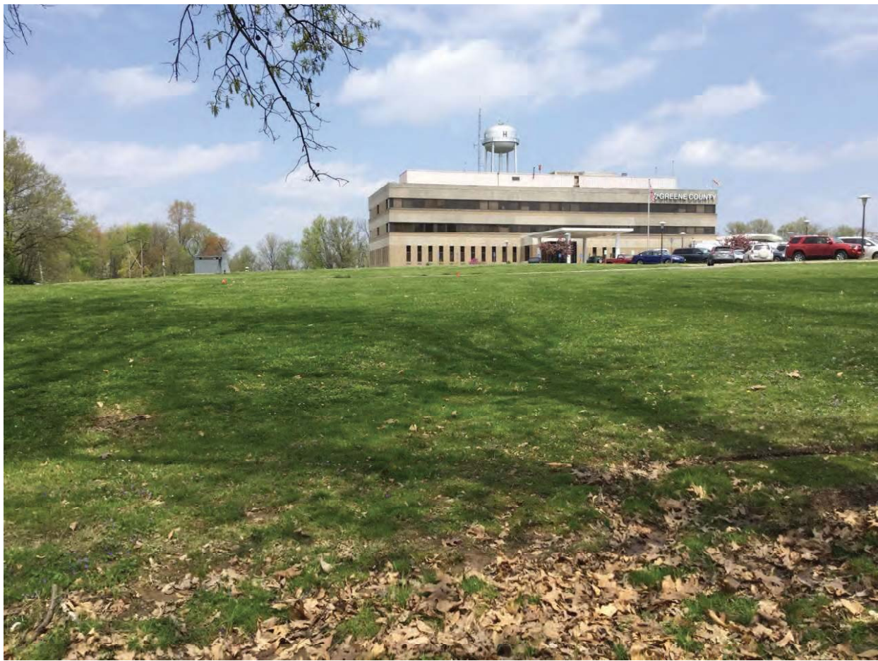
43. Looking north towards Greene County General Hospital from 3N1
