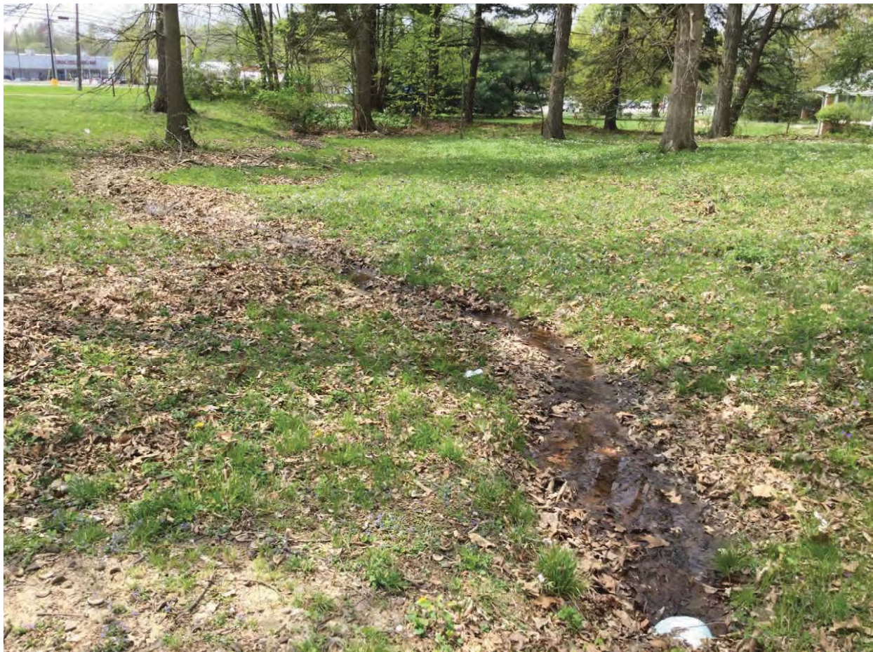
40. Looking southeast from culvert along UNT 6
