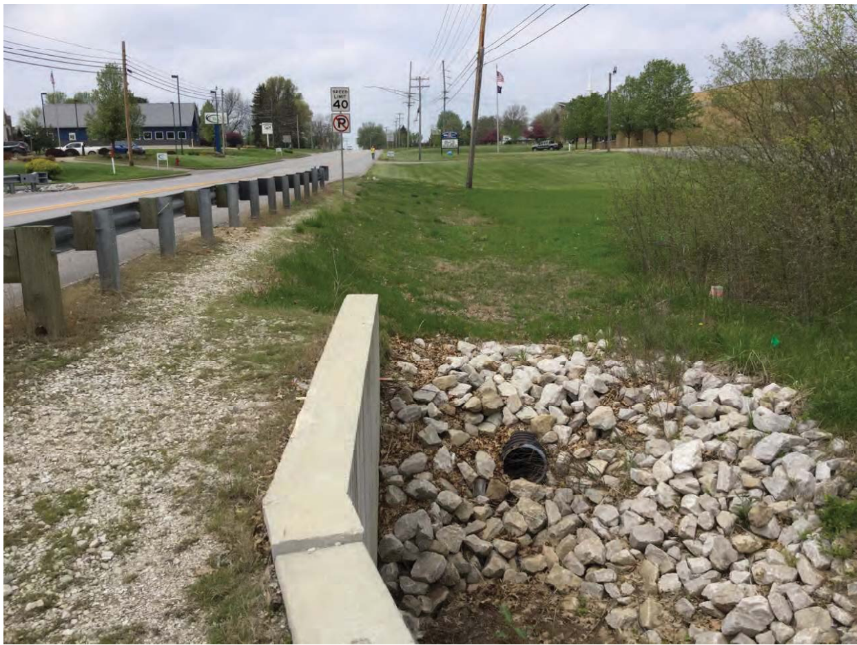
29. Looking west along SR 54 towards culvert that outlets into UNT 4
