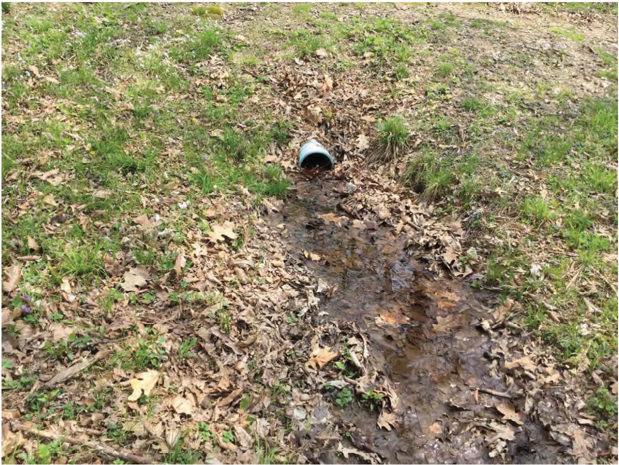
41. Looking northeast at culvert outlet forming UNT 6
