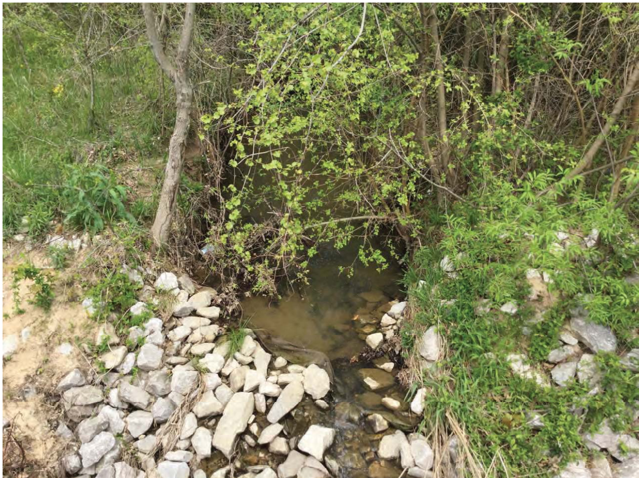
28. Looking north towards UNT 4
